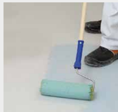
Preparation: Prime floor
