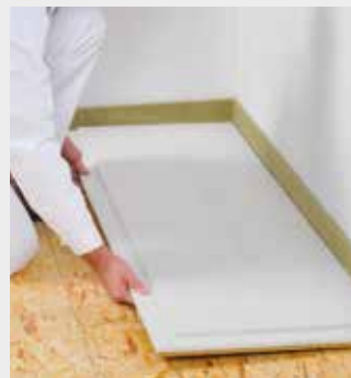
Install the fermacell Flooring Element
