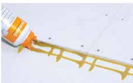
Glue bead at the edge of the board
