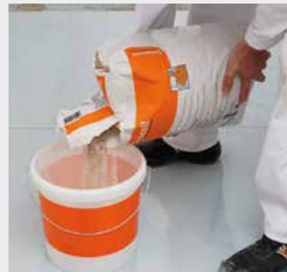
Mix in clean container: 6.5 l water/ 25 kg bag
