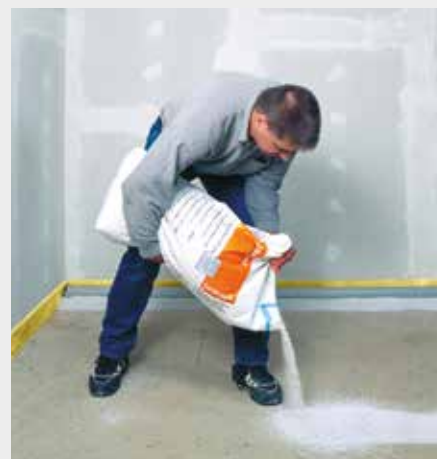
Preparing the area to be levelled
