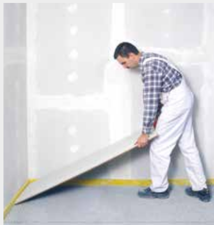
Lay fermacell Flooring Elements
