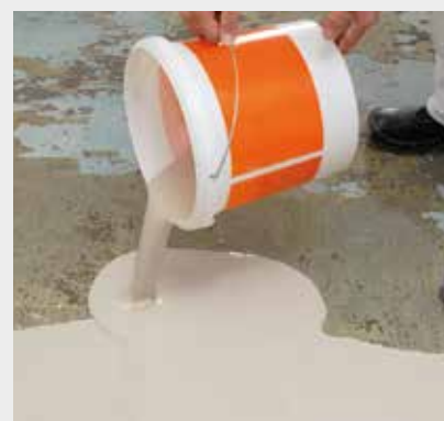
Pour out self-levelling compound and level off
