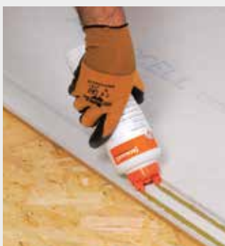
Apply the fermacell Floor Glue to the shiplap joint
