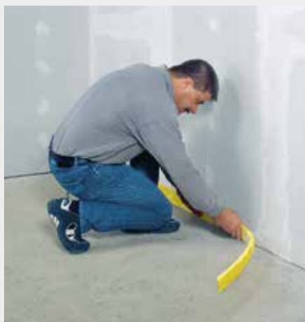
Fitting the perimeter strips
