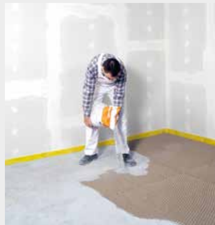
Apply fermacell Honeycomb Infill
