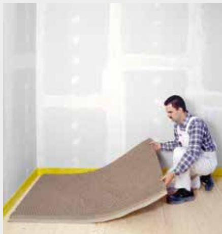
Lay fermacell Honeycomb System
