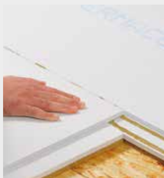
Glue the elements to ensure fully bonded
