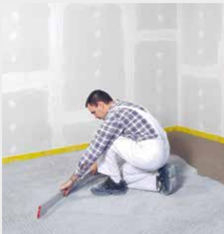
Level out fermacell Honeycomb Infill
