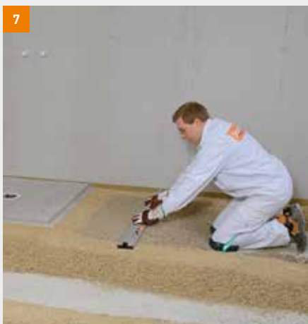
Fill in between the levelled edges and level out.
